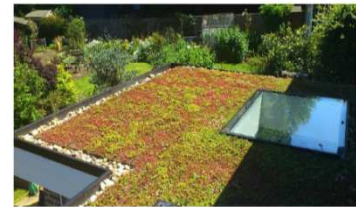
7 Example of a green roof system
